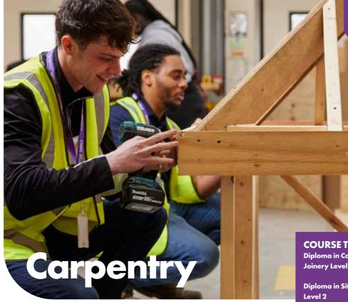
Carpentry and Joinery are both construction trades. Joiners 'join' wood in a workshop, whereas Carpenters construct the building elements on site. Carpenters will install the products made by Joiners, and construct features like the roof trusses, joisted floors and stud-work for partitioning the building.
